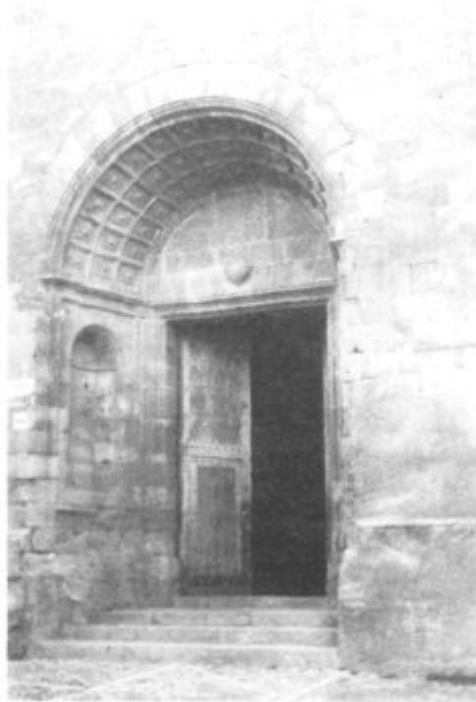
CONVENTO DE SAN BERNARDINO PORTAL PRINCIPAL
