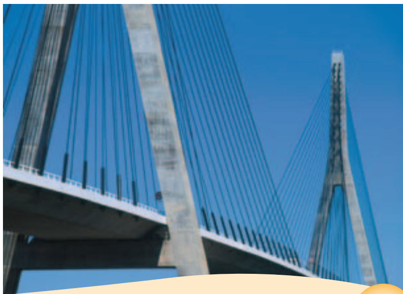
Bridge over the Guadiana river linking Spain and Portugal, a project assisted by the Interreg programme
