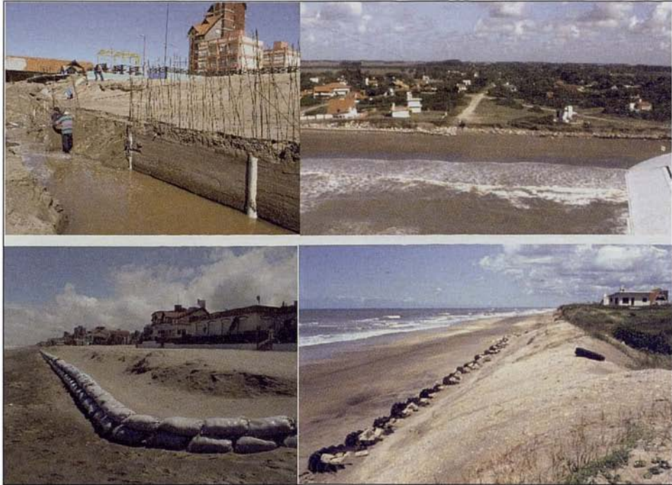
Fig. 7. Alternativas de defensa costera: muros, pedraplenes, bolsas de arena, ruedas de tractores. Fig. 7. Coastal defence alternatives: seawalls, ripraps, sand bags, truck wheels.
