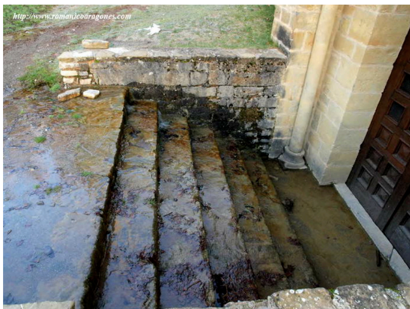
Figure 10. San Adrián de Sasabe, descending entrance stairs (Photo: © Antonio García Omedes).
