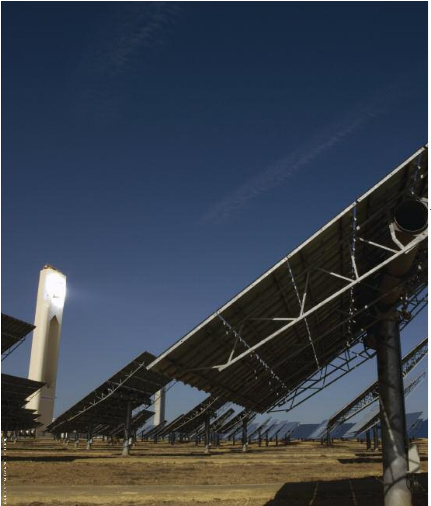
image THE PS10 CONCENTRATING SOLAR TOWER PLANT IN SEVILLA, SPAIN, USES 624 LARGE MOVABLE MIRRORS CALLED HELIOSTATS. THE MIRRORS CONCENTRATE THE SUN'S RAYS TO THE TOP OF A 115 METER (377 FOOT) HIGH TOWER WHERE A SOLAR RECEIVER AND A STEAM TURBINE ARE LOCATED. THE TURBINE DRIVES A GENERATOR, PRODUCING ELECTRICITY.
