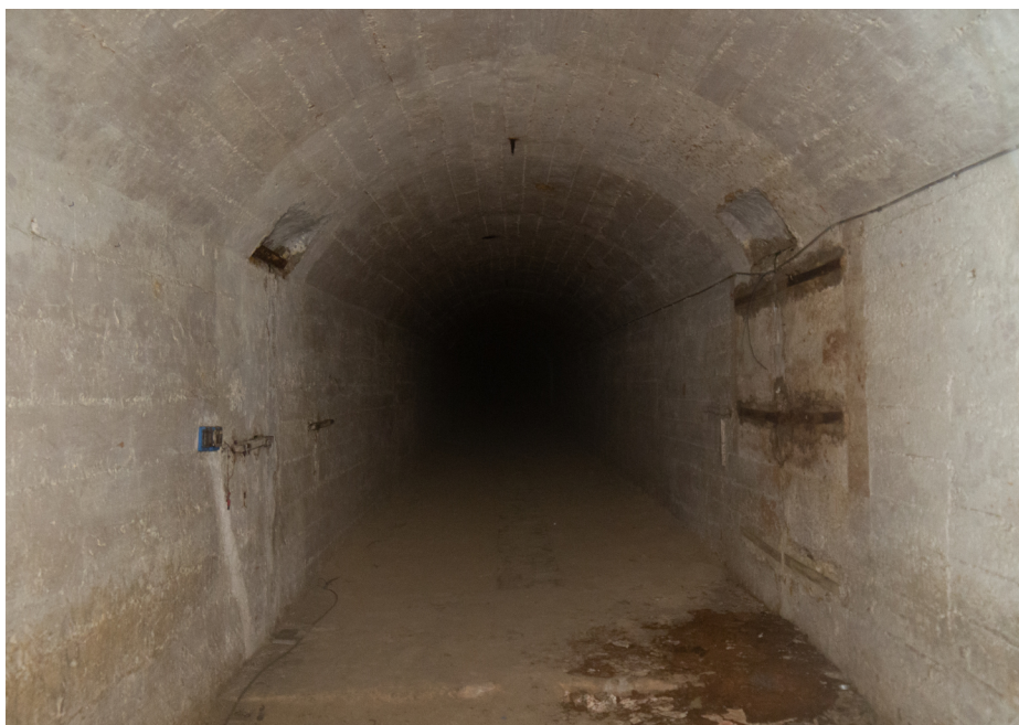
Figura 4. Interior del refugi del Quarter General Luque (Font: Alexandre Luis)
