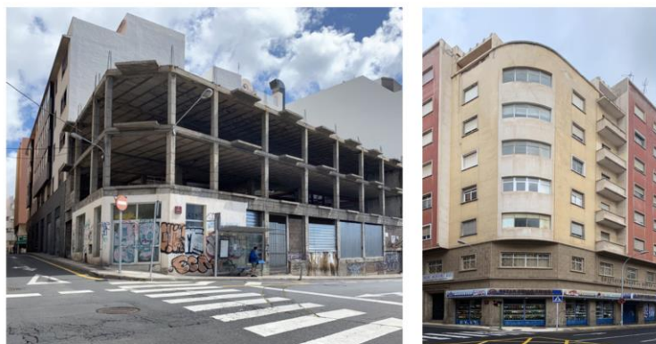
Fig. 1. Symptoms of the housing crisis in Santa Cruz de Tenerife. Left: unfinished and abandoned construction of a building. Right: vacant housing in bad physical condition. Own photos.
