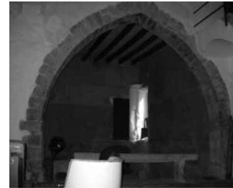
Fig. 15. Arc ogival a Can Monroig
