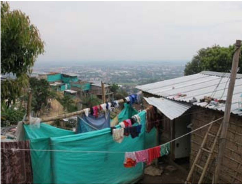
The community of Alto Napoles says that they have installed their own electrical systems and water and waste systems.
